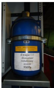
→ Hydraulic Accumulator for Emergency Fast Operations
